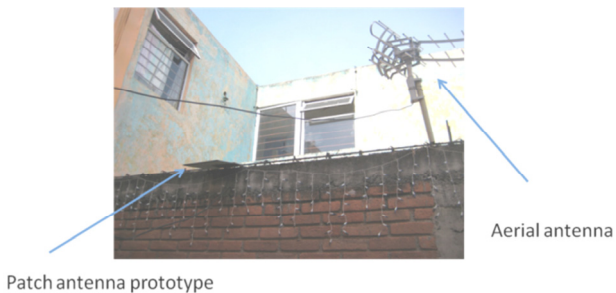
Fig. 15. Location of the antennas used on a house roof in Morelia, Mich.
